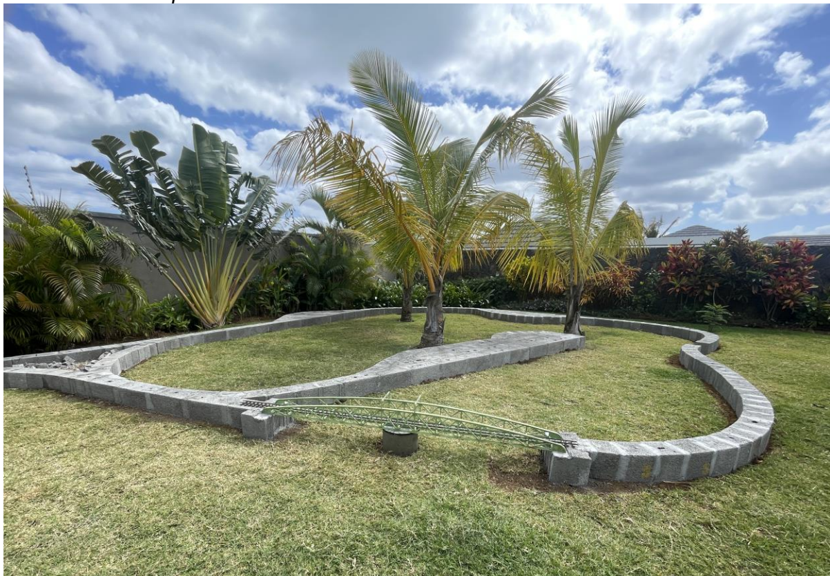
Foundations: breeze blocks
