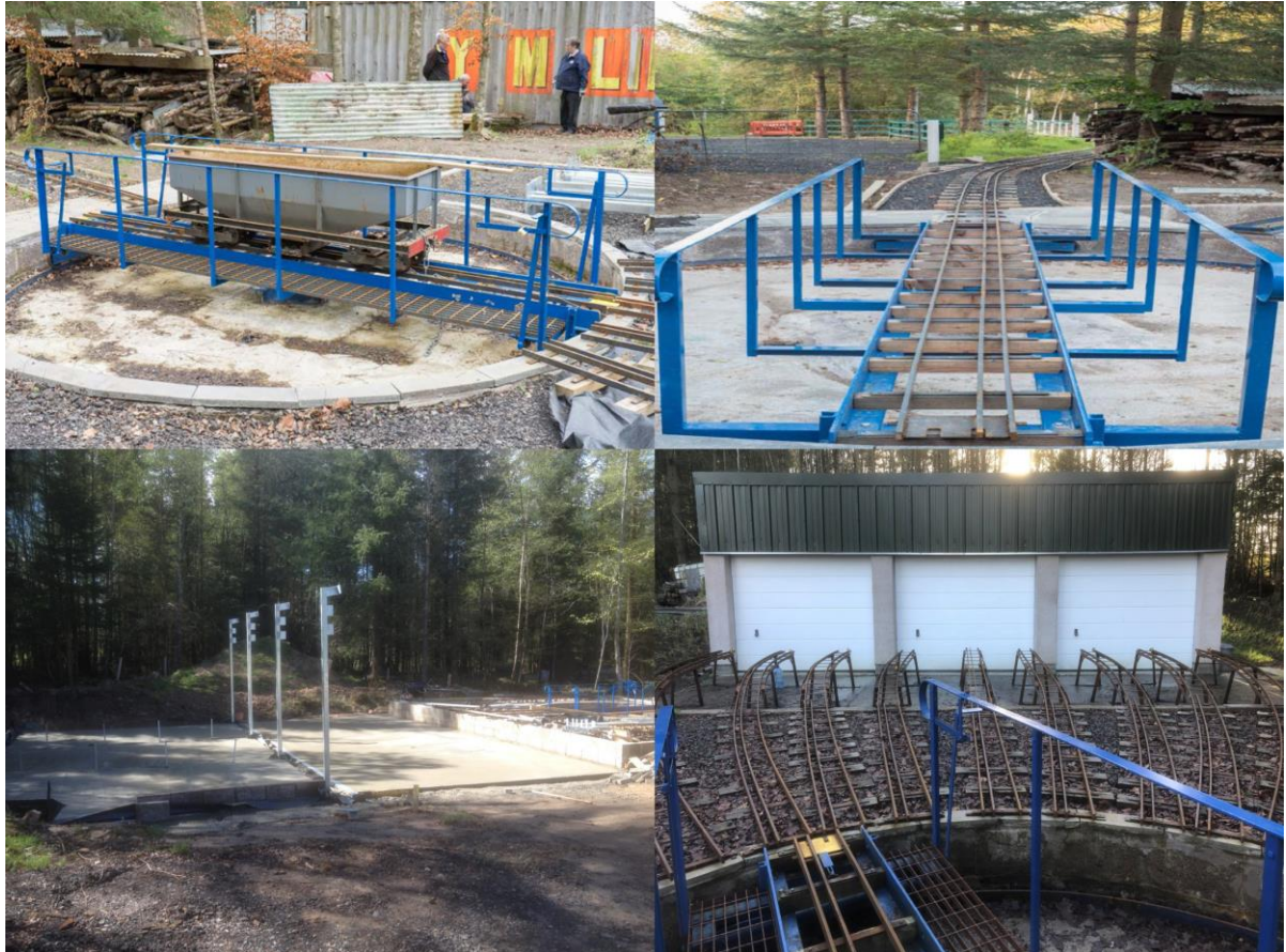
One of two turntables and steaming areas. There are also two unloading areas.
