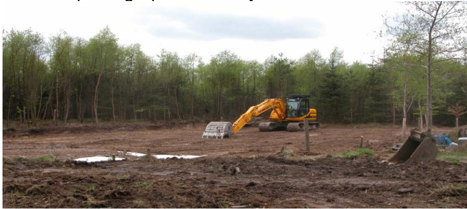
Site clearing for the workshop
