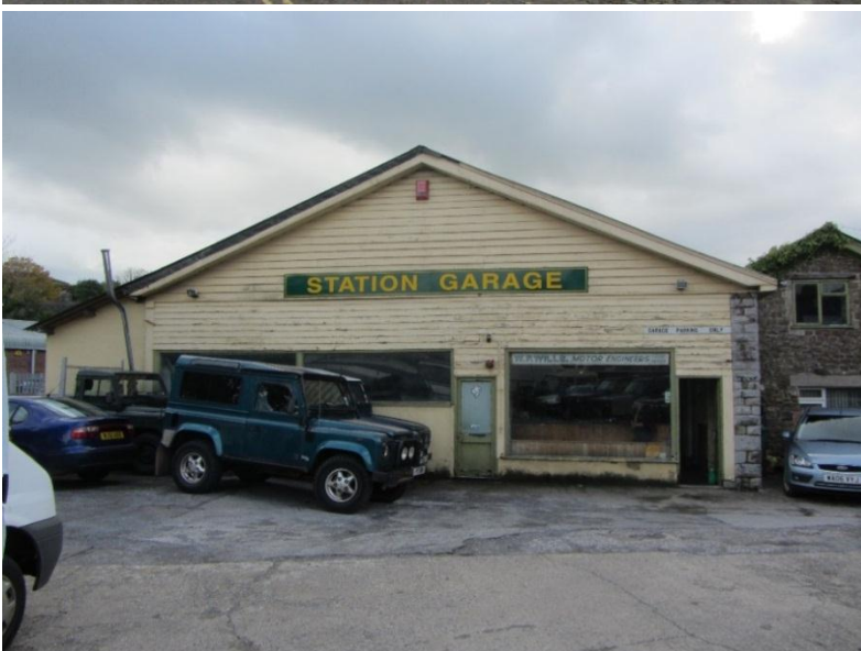
Brunellian style roof and the station building October 2014 And this???? I don't think so. Not sure this building should win any awards for heritage preservation!
